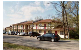
Osage Ridge Apartments
