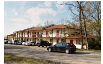
Osage Ridge Apartments
