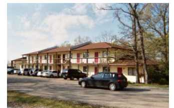
Osage Ridge Apartments
