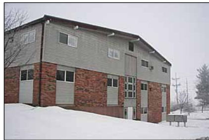
NOW: LVC as it appears today. Unable to salvage the siding and entryway doors, we are replacing with concrete Hardi-products and commercial low-E Glass entryways.
